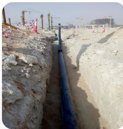
MAIN IRRIGATION HDPE PIPE
