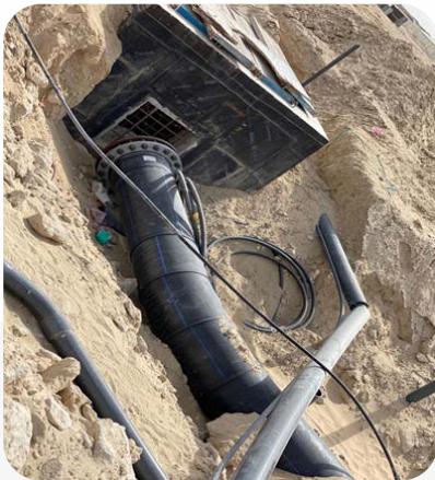
MAIN IRRIGATION HDPE PIPE
