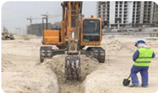
EXCAVATION FOR POTABLE WATER
