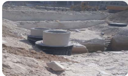
SEWERAGE MANHOLES
