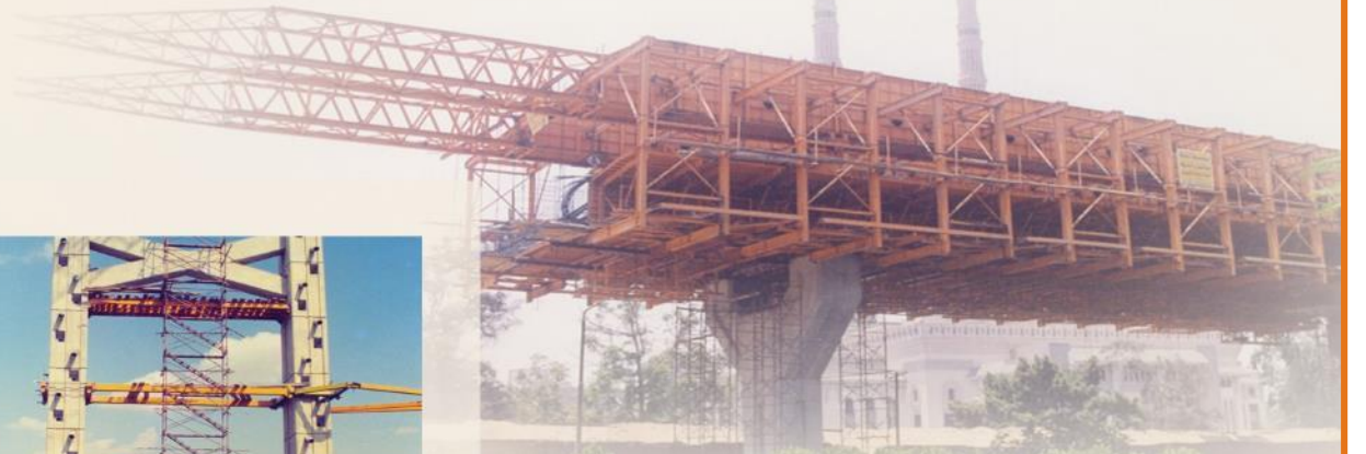
Advancing Shoring System, 6 th of October Viaduct
