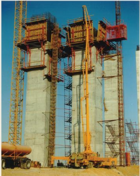
Climbing Formwork, Mubarak Peace Bridge
