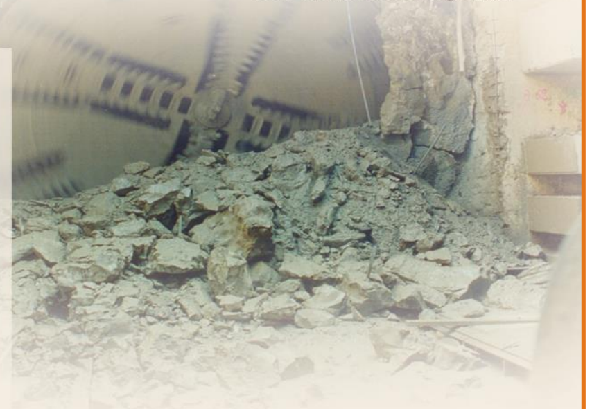
TBM at the Receiving Shaft
