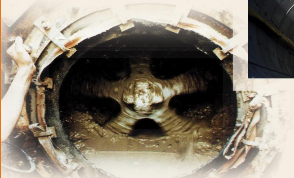
600 mm Reaching the Receiving Shaft
