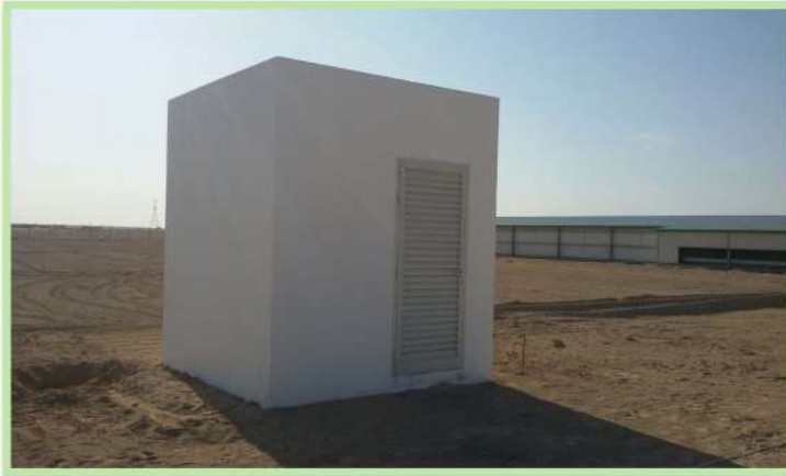
Electrical Substation for Broiler Houses
